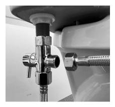
5. Connect the metal hose supplied with the bidet to the open side of the t-valve.
