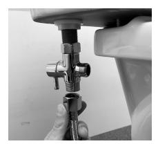
4. Attach the water supply hose (attached to the water shut off valve) to the bottom of the t-valve.
