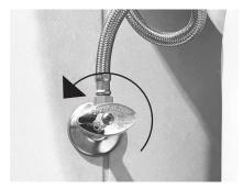
13. Slowly turn the water supply valve open. Check for leaks as the valve opens. If leak occurs, turn off the water supply and tighten the connection properly.
