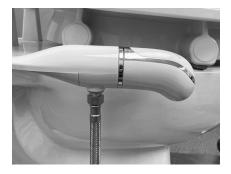
Connect the hose from the t-valve to the bidet attachment and tighten.
